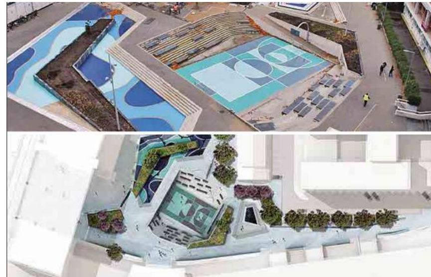
Water Square, Rotterdam, NL
